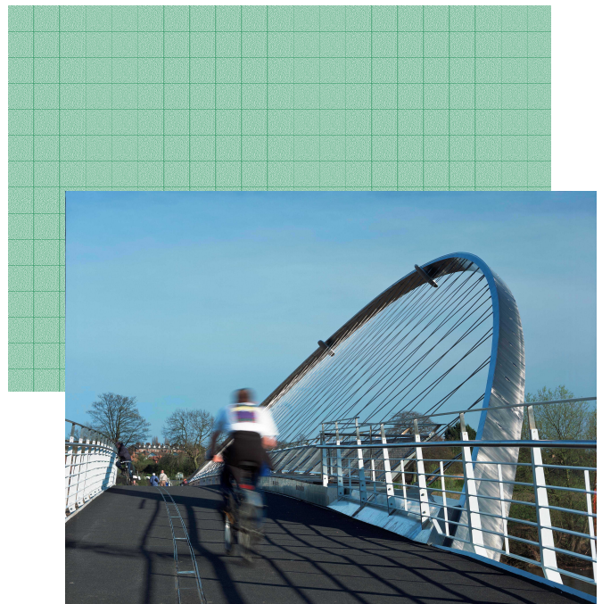
Millennium Bridge, a pedestrian and cycle bridge which forms part of the cycle and pedestrian network across the City. Linking Fulford and South Bank area
